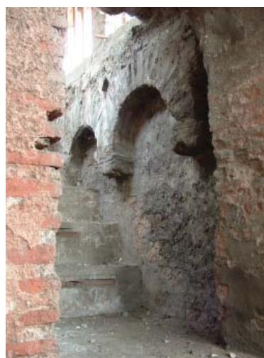
Fig. 11. Staircase connecting the martyrium to the basilica
