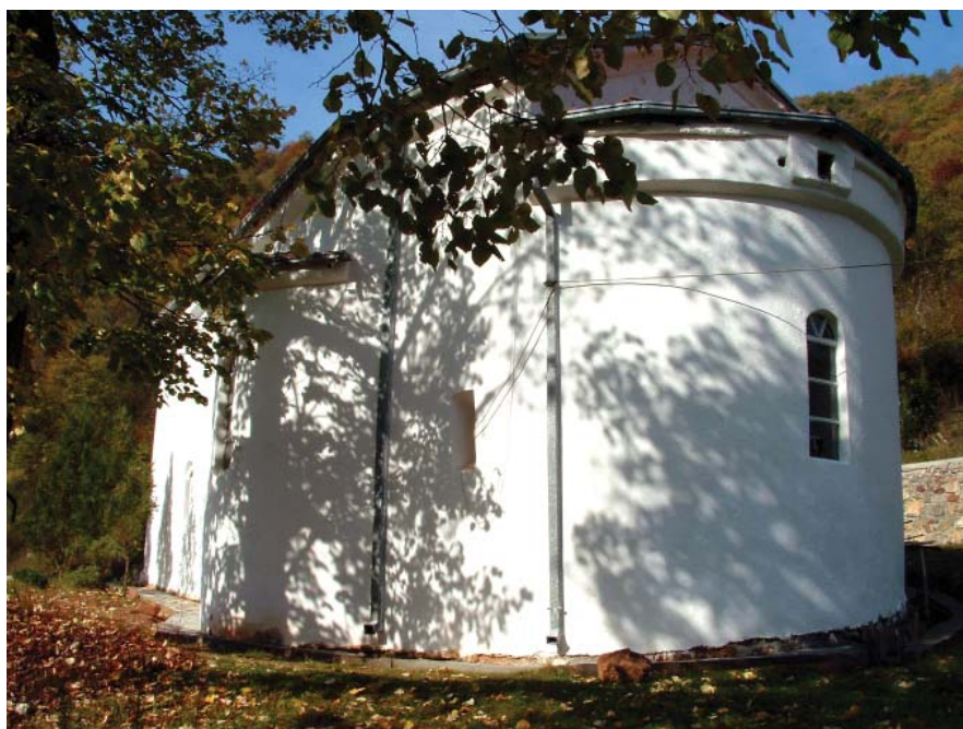
Fig. 30. Matejevac, Church of St. John, the southeastern view
