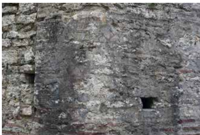
Fig. 11. Plastering of the eastern facade with imitation of masonry in Great Basilica of Butrint at the Ionian coast, end of the 10 th century, Albania (photo by S. Maltseva)
