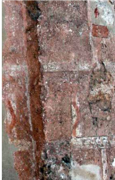
Fig. 9. Traces of plaster with imitation brickwork on the eastern facade in Zemen, mid-11 th century. Bulgaria (photo by S. Maltseva)
