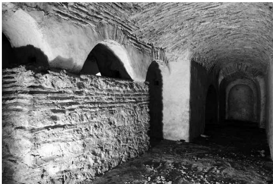
Fig. 1 Enveloped columns in the substructure of the church of Maria Eleousa (Nuran Nar)
