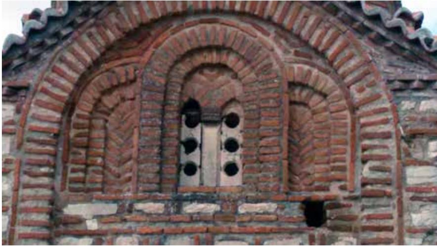
Fig. 4 Photo Holy Trinity church, detail of scalloped bricks. Photo E. Kodheli
