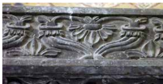
Fig. 4 Hagia Sophia, wooden casings of tie-beams on gallery above narthex, photo author
