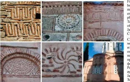
Fig.6. Collage: brickwork meanders, several examples, photo: Rémi Terryn; author of the collage: Jasmina S. Ćirić Сл.6. Колаж: меандер
