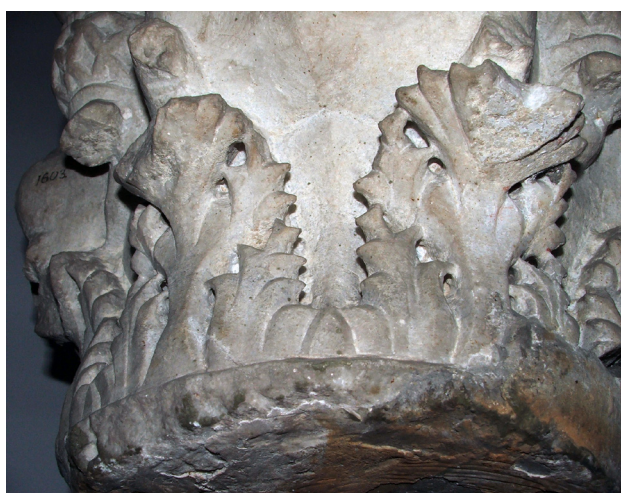
Fig. 10. Figural double zoned capital in Composite order, cat. Nr. 2, detail of acanthus foliage, spaces of calathos between the leaves and the soffite band in profile;
