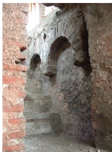
Fig. 11. Staircase connecting the martyrium to the basilica
