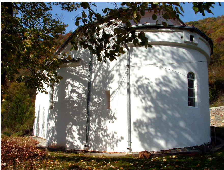
Fig. 30. Matejevac, Church of St. John, the southeastern view
